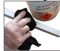
Degrease with solvent
