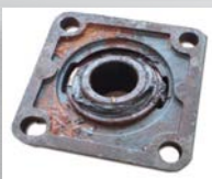
Clean off rust & debris with a wire brush
