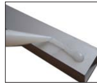
Dispense bead of adhesive, do not spread
