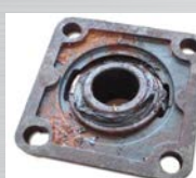
Clean off rust & debris with a wire brush
